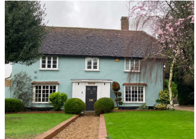
Figure 59: Older building within the character area featuring best practice exterior finishes.
