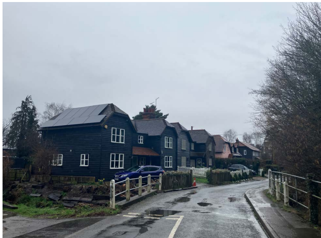
Figure 79: Row of terraced housing with jerkin head roofs and black weatherboard exterior finish.
