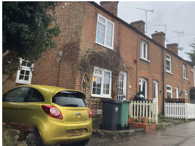
Figure 44: On-plot parking to the side of a dwelling.
