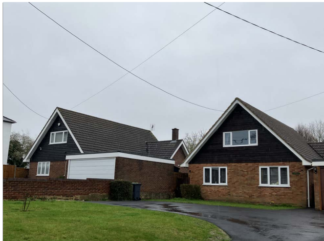
Figure 63: Example of appropriate scale and massing of a two properties between Wright's Green and Mott's Green.
