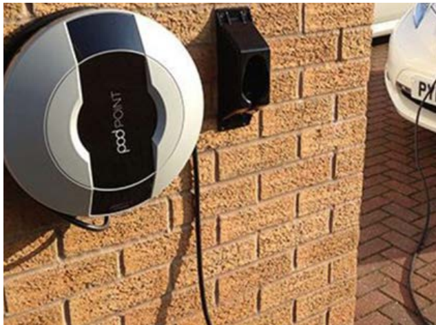
Figure 43: EV charging for private on-plot parking (elsewhere in the UK).
